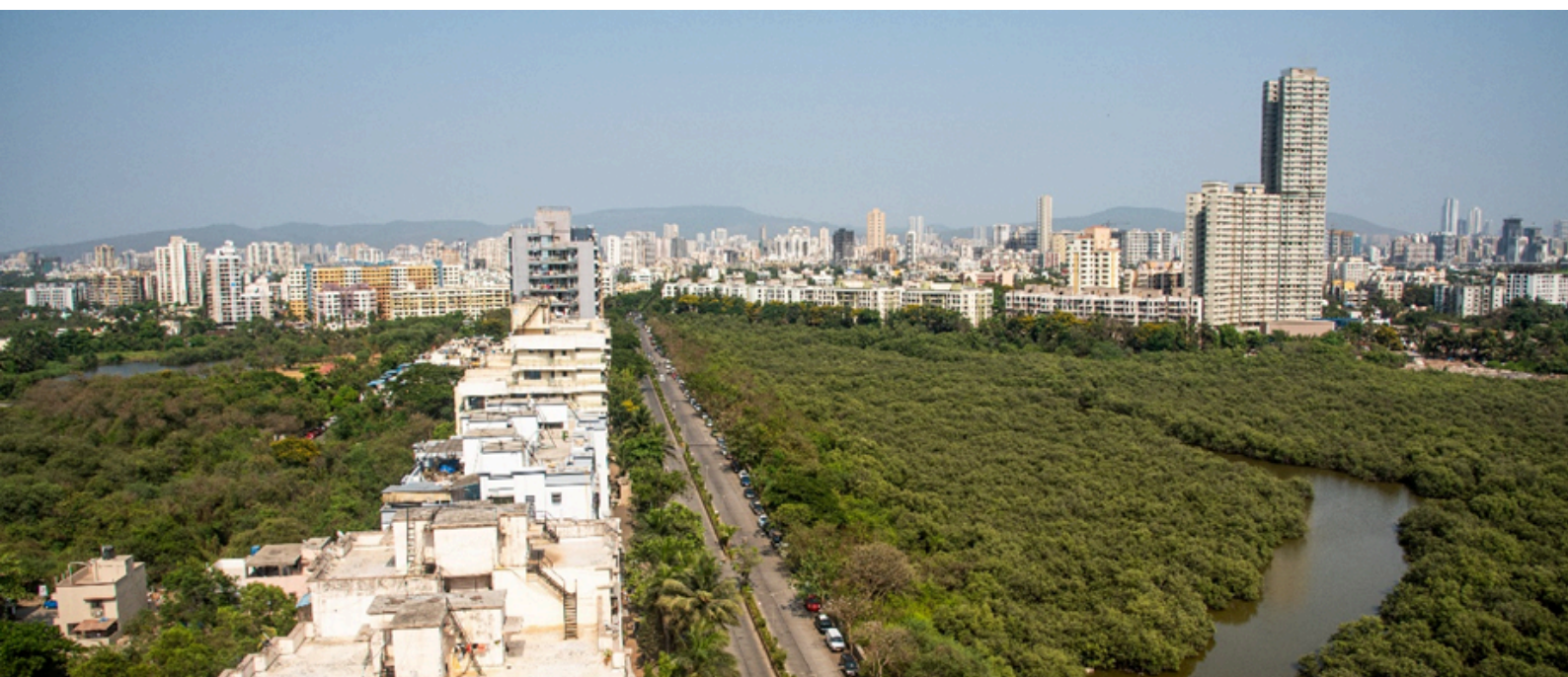
Aerial view of roads and mangroves in Mumbai. Photo by Parikh Mahendra N/Shutterstock.
