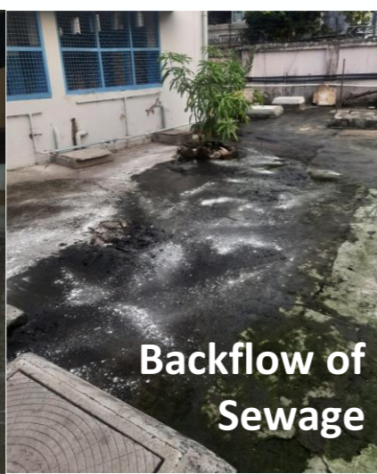
Flooding at LFC 07 Nov 2021
